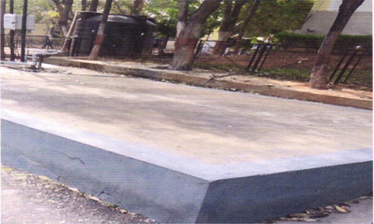
Water harvesting Pit
