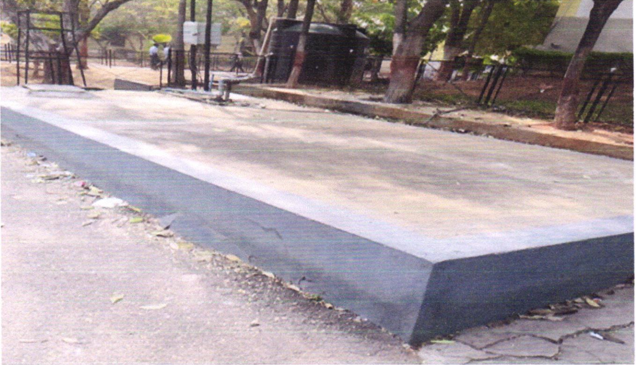
Water harvesting Pit
